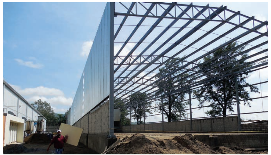
This is the steel frame of the expanded metal-working operations at the Zapopan plant.
